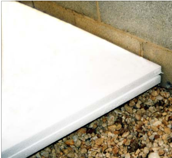
A health promoting building regulates the temperature and moisture content of the indoor air to enhance circulation and prevent condensation.
